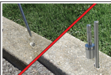
Drill a 3/4" hole & insert base
